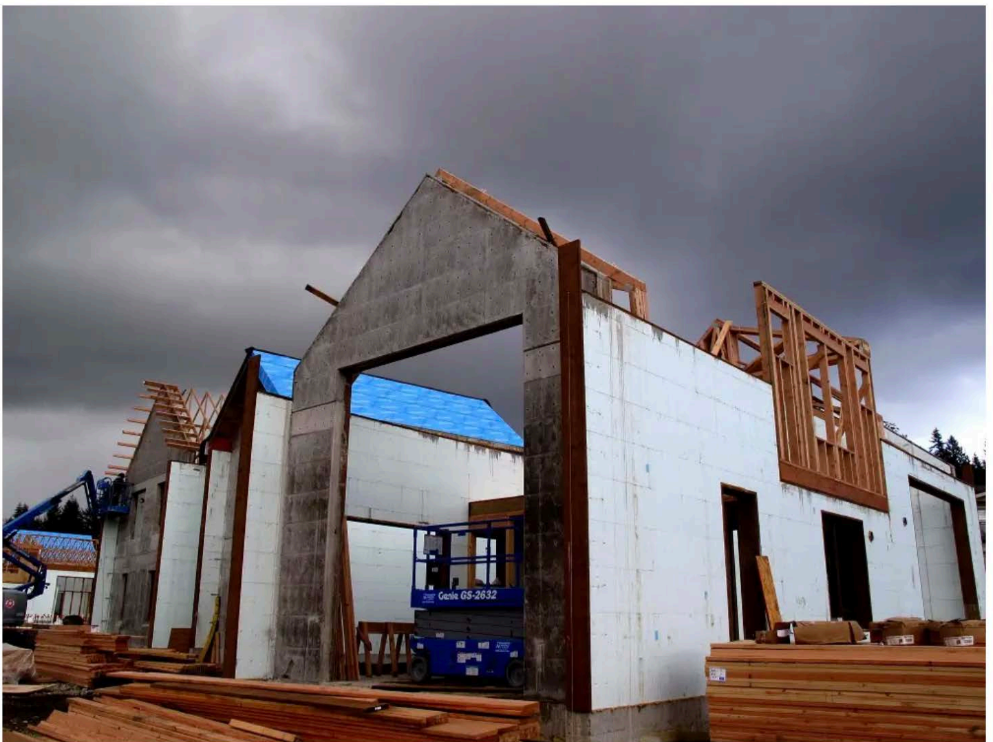
Photo courtesy of Clark Construction, LLC
