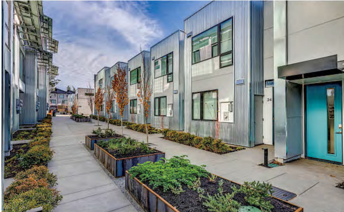
The Walk is the first multifamily project on Bainbridge Island to be registered as a Living Building Zero Energy Project.
